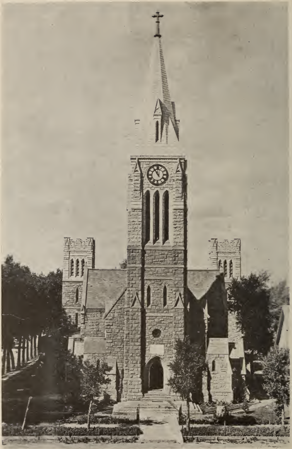
SAINT MATTHEW'S CATHEDRAL, LARAMIE The two towers have recently been completed
